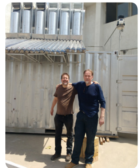
Solar-Polar’s Michael Reid and Robert Edwards with the innovative system following installation on a rooftop in Ahmadabad.
